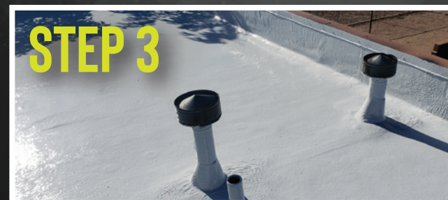
APPLY UV PROTECTIVE COATING
