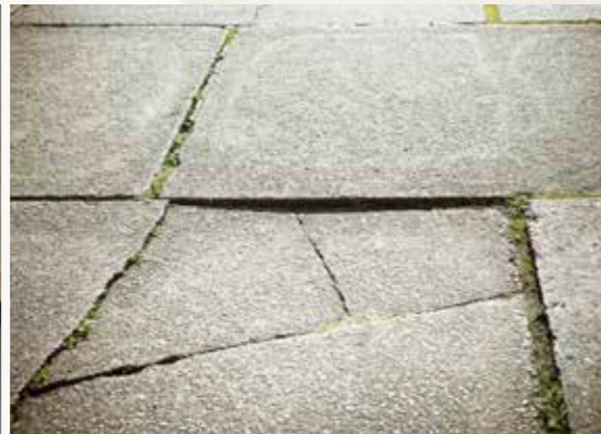
Concrete Lifting
