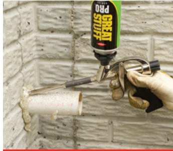
PVC pipe penetrations
