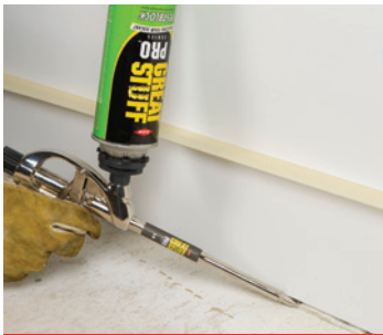
Under baseboards and attic hatch frames
