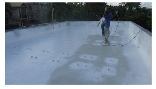
ExpandoThane is to be applied by a Hot High Pressure Plural Component Machine
