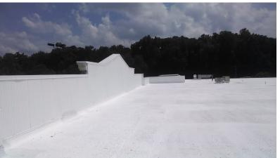
Silicone Seal 3000 Roof Coating is a single component spray grade high solids VOC free material available in white, and light or dark grey colors.
